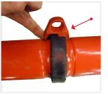
Place the second housing over the bolt and turn the nut fingertight on the bolt. Then place the second bolt and tighten it finger-tight.
